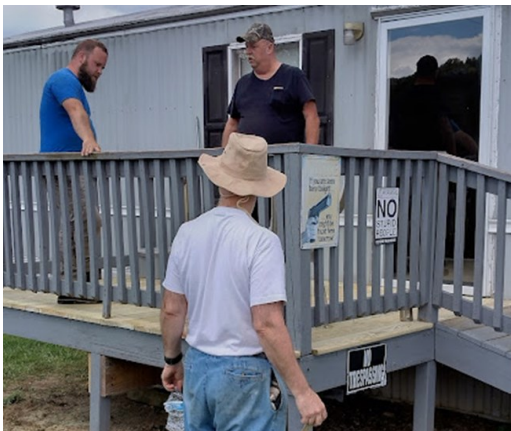
The 2nd project was replacing the boards on the deck and reinforcing them making it sturdier.
