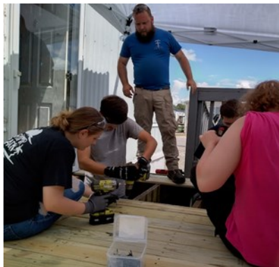
The 2nd project was replacing the boards on the deck and reinforcing them making it sturdier.
