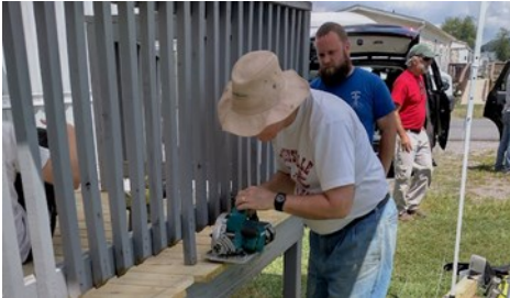
The 2nd project was replacing the boards on the deck and reinforcing them making it sturdier.
